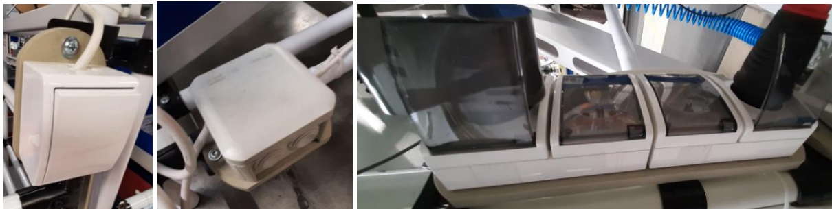
Fig. 7 – Photo depicting a finished solution in the production area
